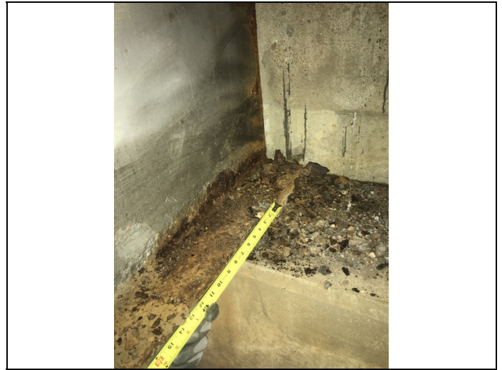
Span 1 bent 1 girder 4 hole in left side of bottom flange at with section loss at bottom of web
