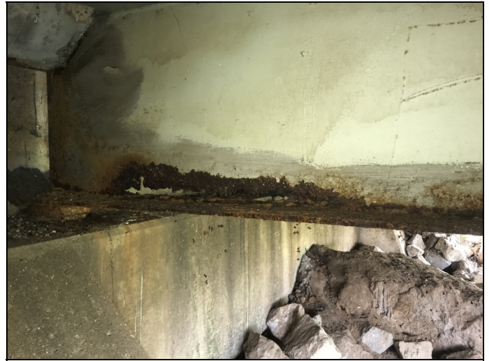
Span 3 bent 4 girder 2 back side of 22" hole in bottom of web
